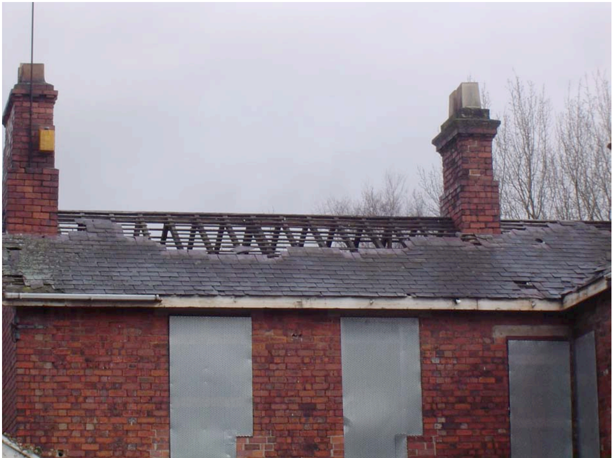
Unsafe building needs repair or demolish
