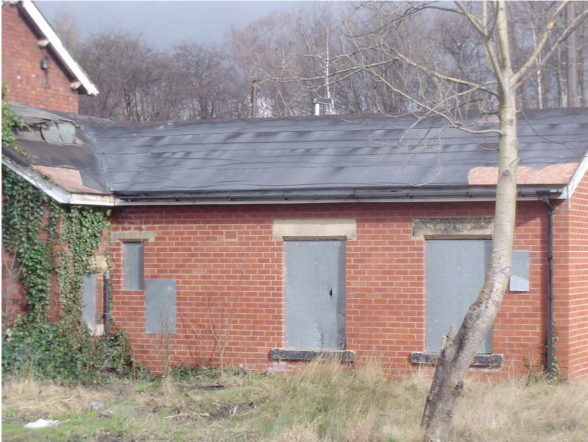
Current Station buildings
