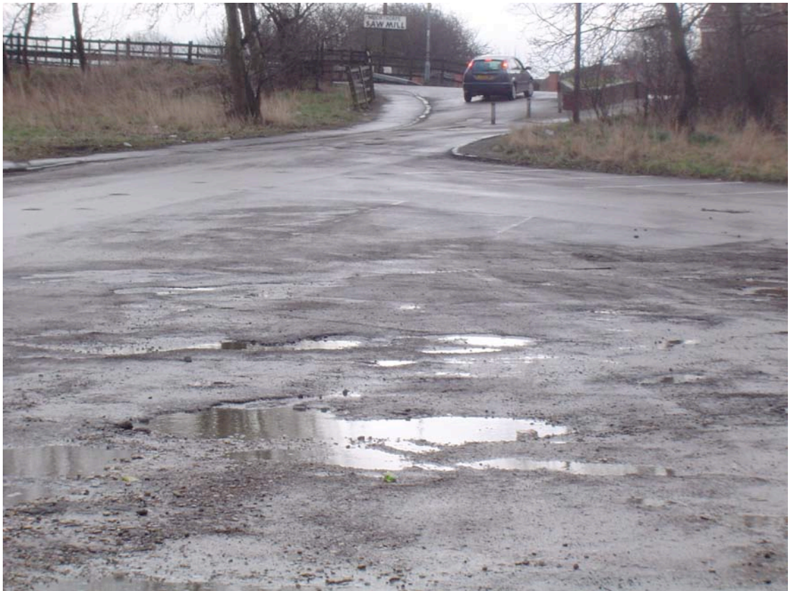
Moorthorpe Station Car Park
